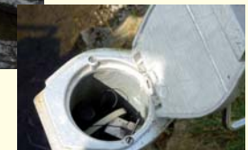
Blick in Pegelrohr
